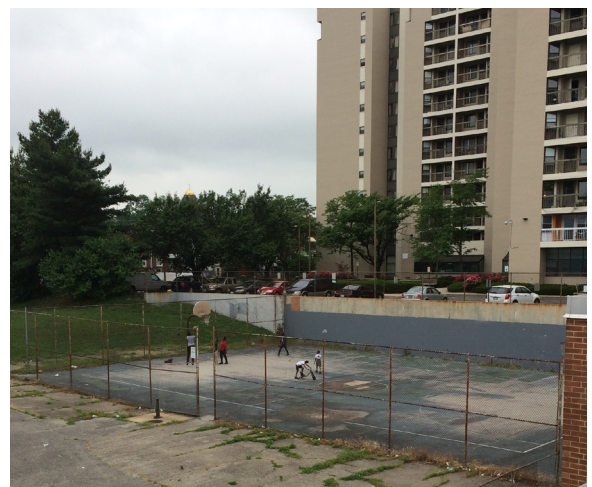
Basketball Court and Retaining Wall
