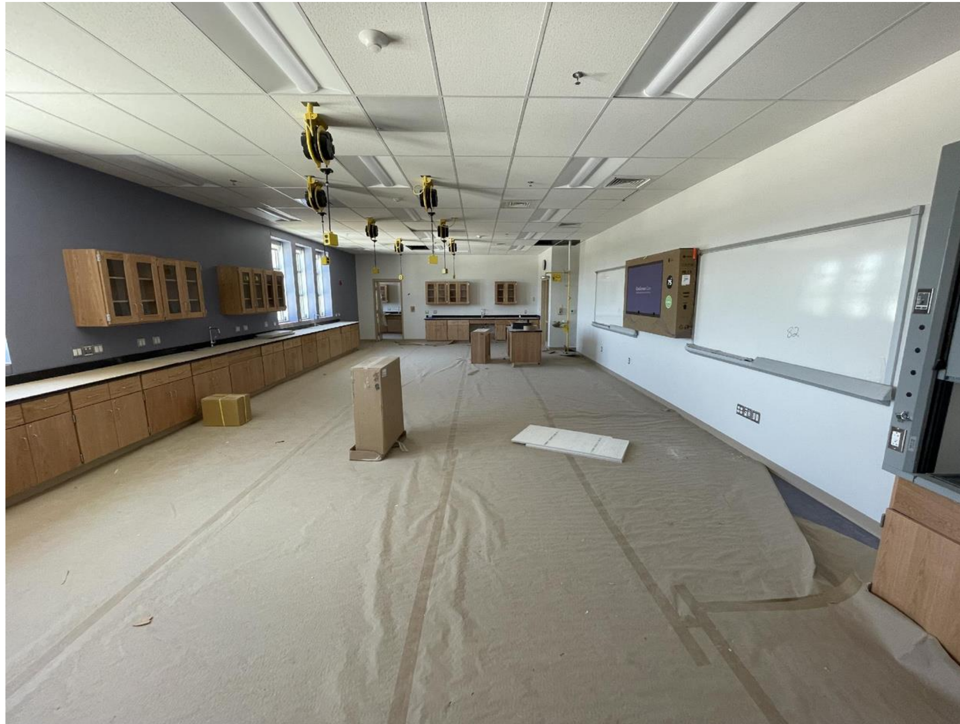
CLASSROOM – All finishes & equipment have been installed
