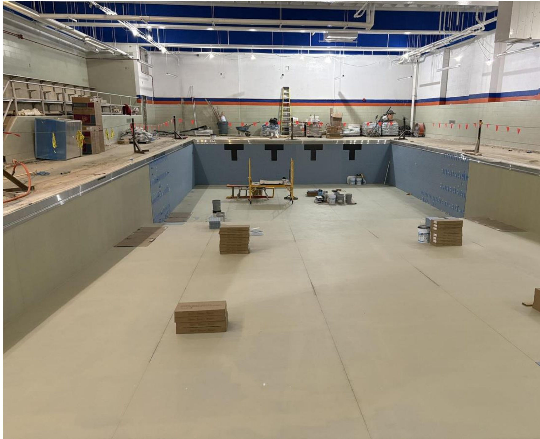
POOL – the pool shell work is complete; tile is being installed & the majority of the work in the ceiling has been completed
