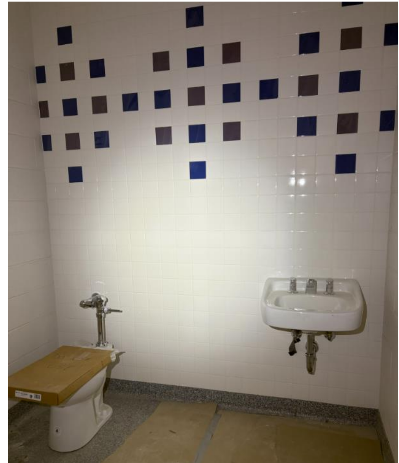
RESTROOM – Flooring, wall tile & plumbing fixtures have been installed.
