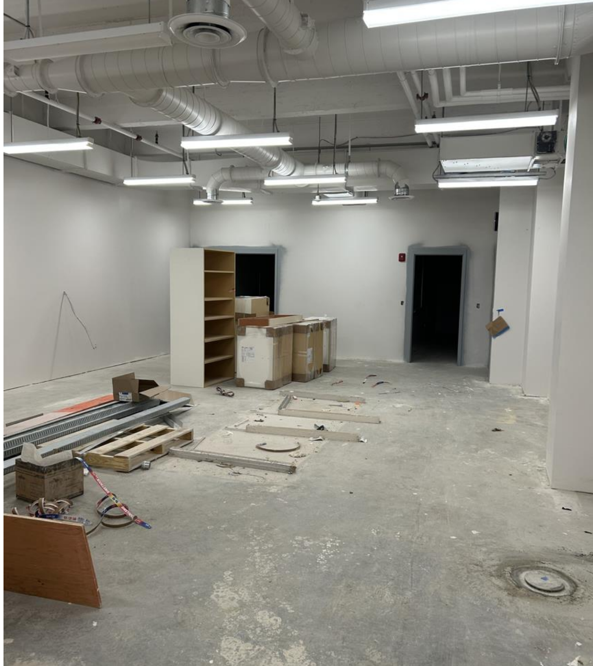
CONSTRUCTION ROOM – This will be the lab portion with exposed ceilings.
