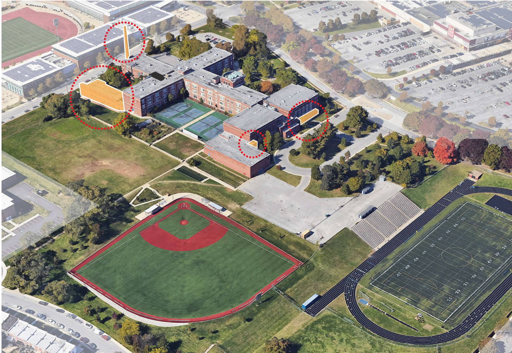
Community Meeting: Construction Kickoff | Frederick Douglass – Briscoe | May 9 th , 2024 baltimore21stcenturyschools.org
