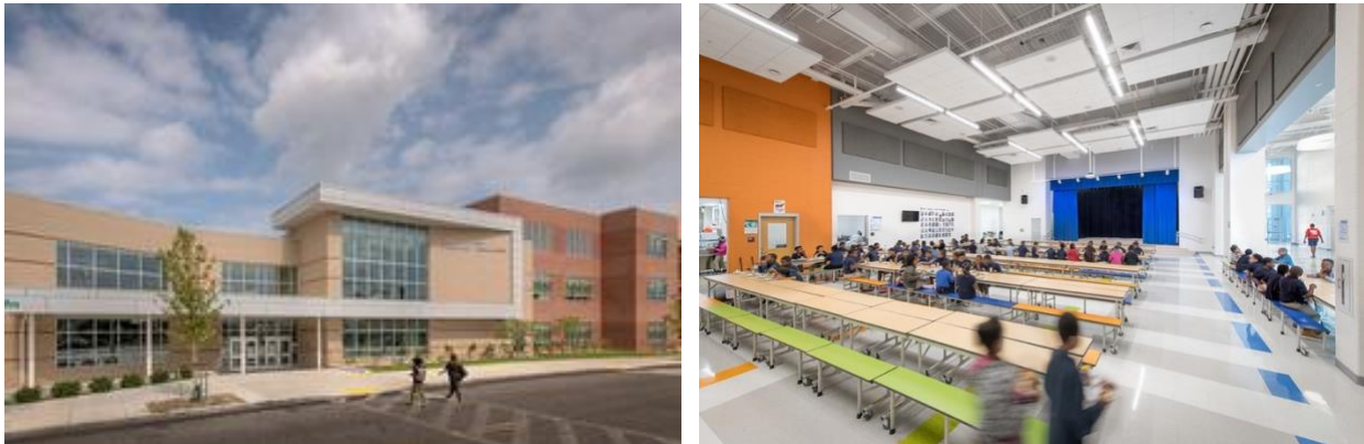
Photos courtesy of Grimm + Parker Architects; Photo credit: Sam Kittner; Fort Worthington exterior and cafeteria
