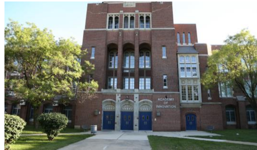
Existing Frederick Douglass High School Building
