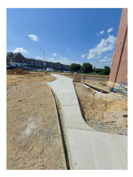
New sidewalk poured (continuation to 32<sup>nd</sup> Street). Staking out for additional sidewalks and paths
