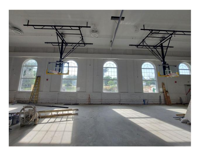
Paint Gym ceiling and walls, install basketball backboards, divider curtain. HVAC trim out
