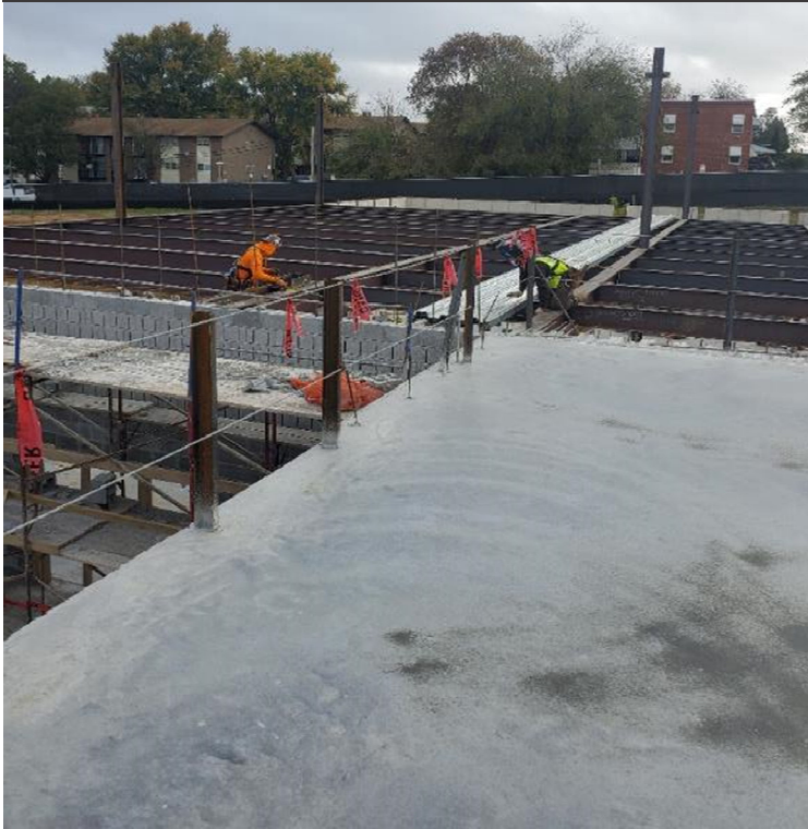
2 nd Level Metal Decking Install
