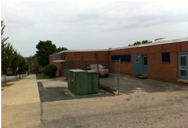
East Service and Loading
