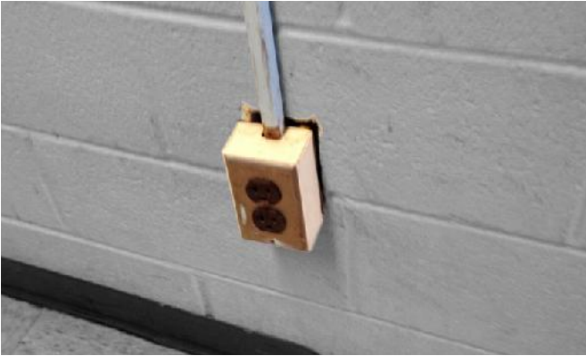
Typical condition of existing electrical receptacles
