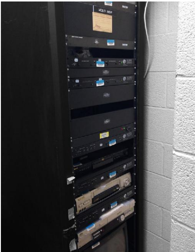
View of existing IT cabinet
