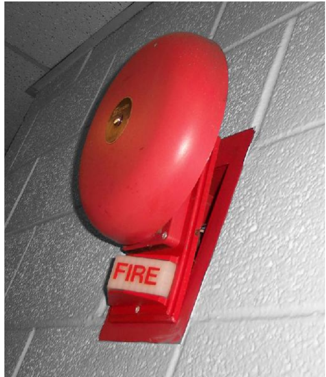
Damage to existing fire safety equipment is evident; updated equipment will need to be installed
