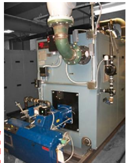
View of one new boiler in Lower Level Mechanical Room
