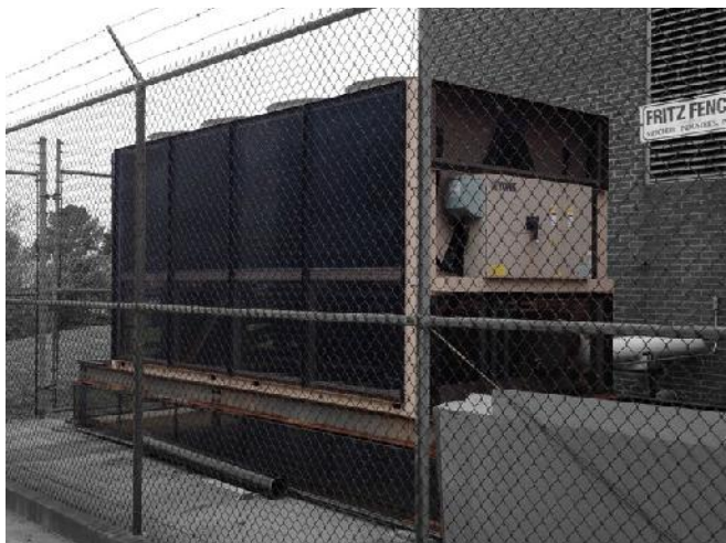
Existing scroll chiller near basement Mechanical Room
