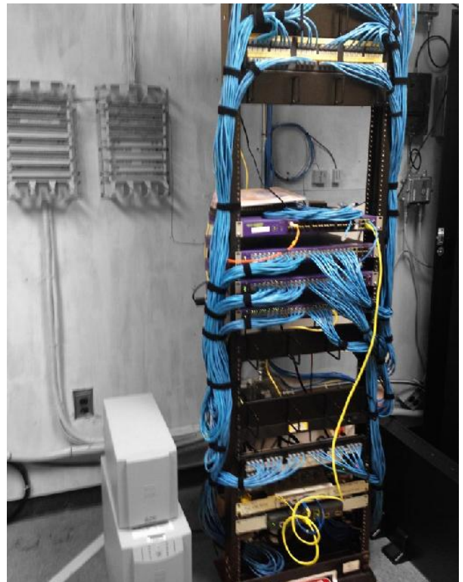
View of existing IT floor rack
