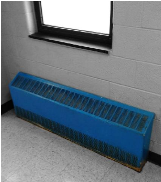
View of existing heating element in hallway
