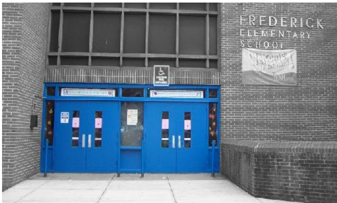
View of existing Main Entry and painted clerestory windows in double-height lobby interior
