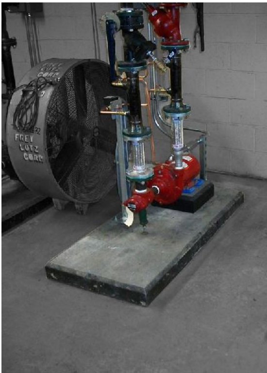
View of new water pump in Mechanical Room
