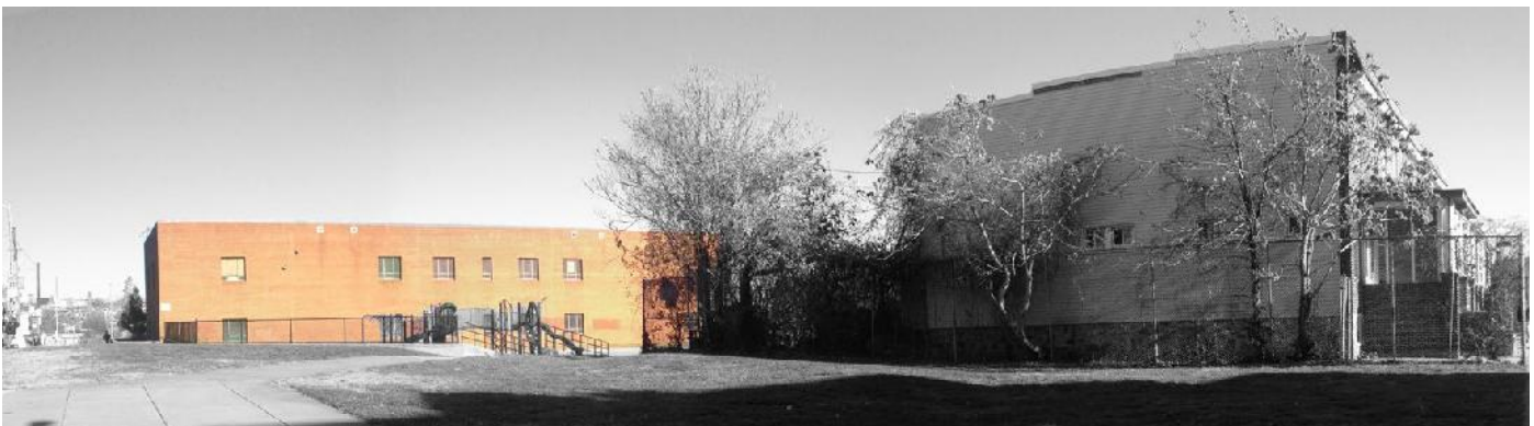
View of Frederick Elementary School from the corner of Frederick and Millington
